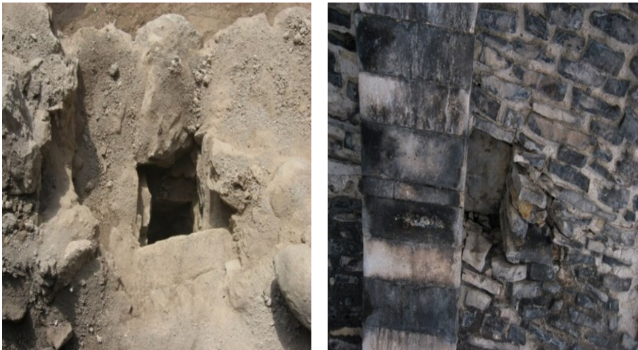
Fig. 9. The view of the skylight from the roof and from the hall. Photo by M. Sargsyan
