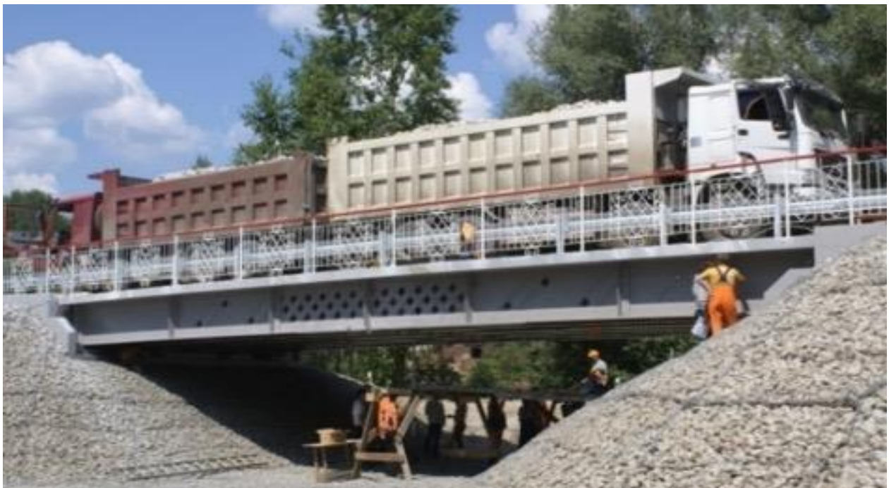
Fig. 2. Static test of the composite span
