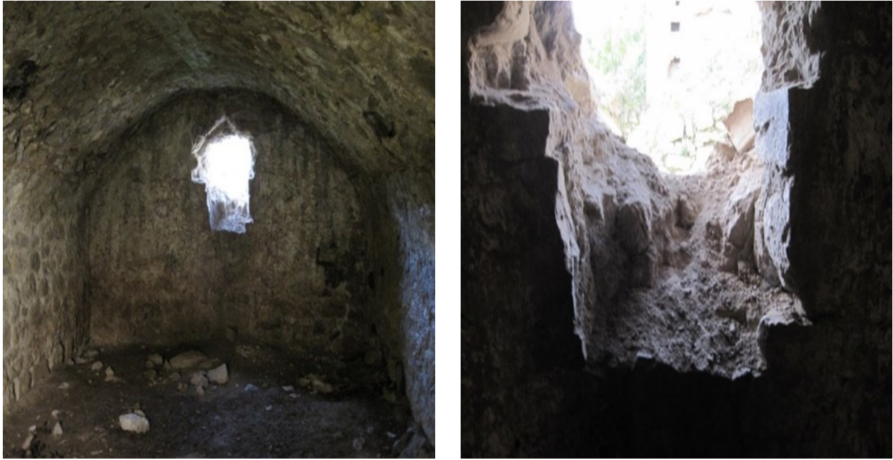
Fig. 11. The niches of the vaulted room in the semi-basement, the exit of the horizontal vault extending from the room. Photo by M. Titanyan
