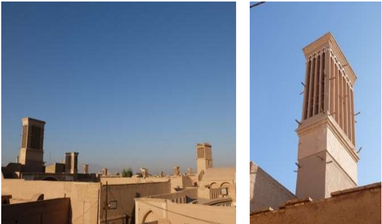
Fig. 3. The historical town of Yazd in Persia and the wind towers. Photo by M. Titanyan
