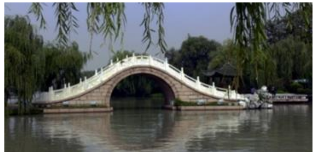
Fig. 9. Moon Bridge in Yangzhou, Jiangsu Province: the ‘ synthesis bridge ’
