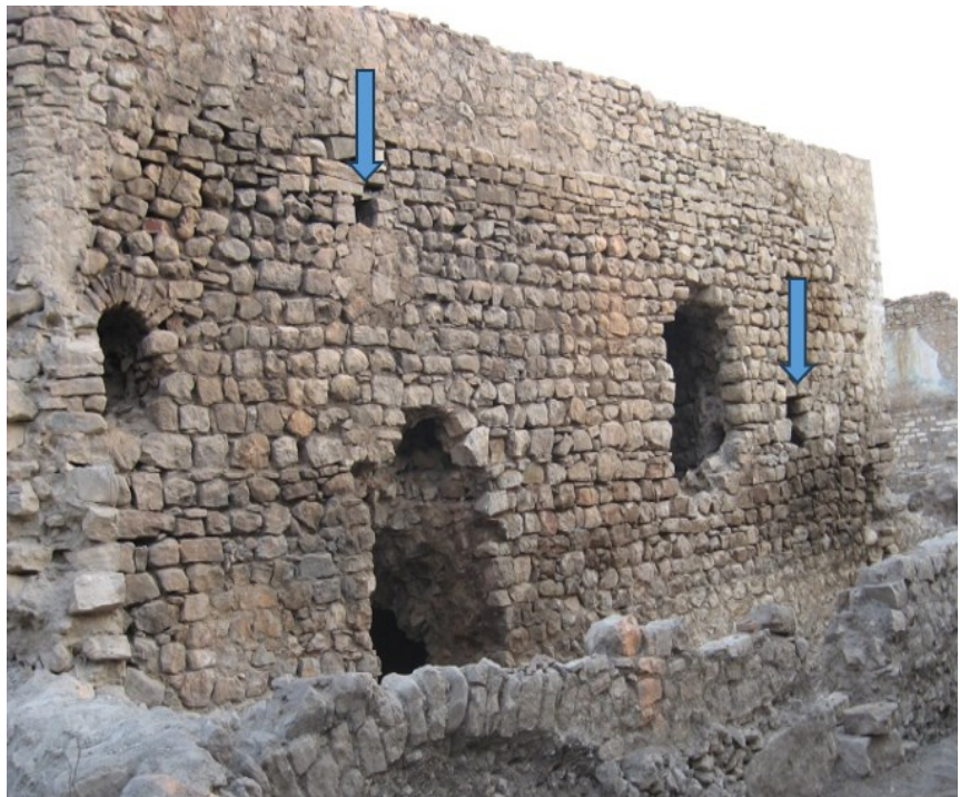
Fig. 7. The first-floor window (left) and the exit of the horizontal well (right) in the southeastern facade. Photo by M. Titanyan
