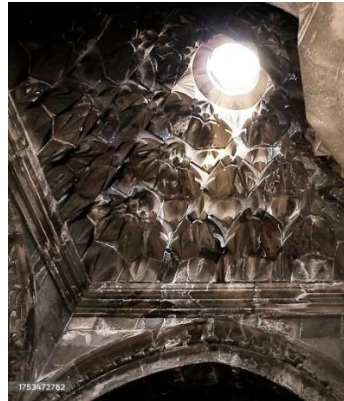
The ceiling of the gavit of Geghardavank
