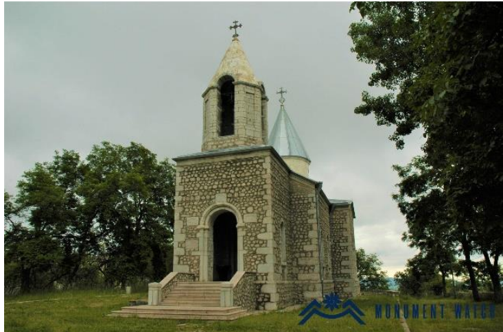
Fig. 3. General view of the St. Hovhannes Mkrtych Church of Shushi from the southwest, 2020, before the war 6
