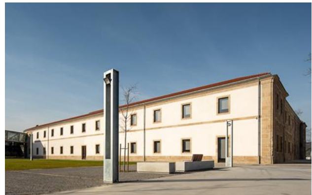
Fig. 17. Back façade of monastery after rehabilitation
