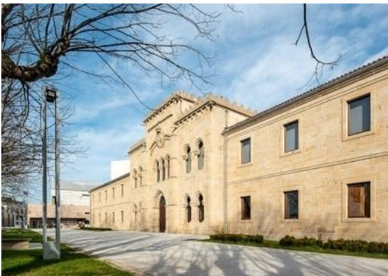
Fig. 16. Front façade of monastery after rehabilitation
