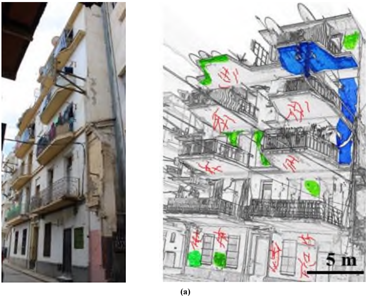
Fig. 7. Mapping of detected anomalies at different inspected surfaces paints: (a) CRAH, (b) CFEM, (c) CLEM, (d) LBB 1, (e) LBB 2, (f) LBB 3
