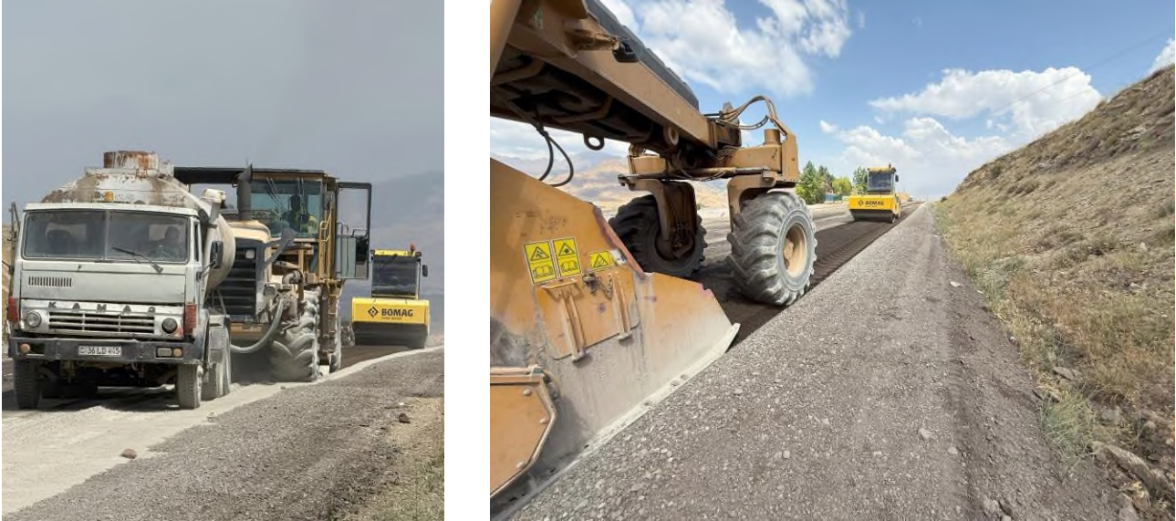
Fig. 5. Full-Depth reclamation and profiling of road pavement
