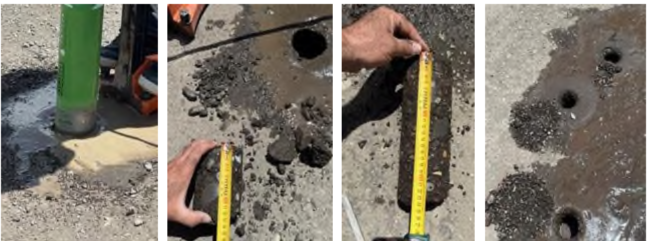
Fig. 6. Core sample extraction
