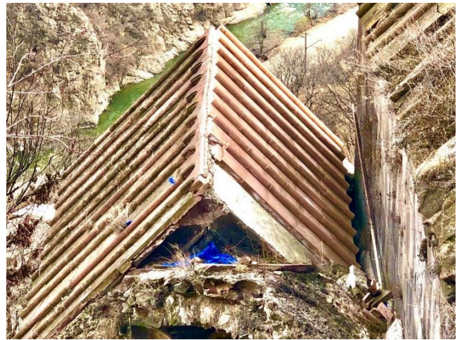
Fig. 5. The bad condition of the Kobayr chapel's roof
