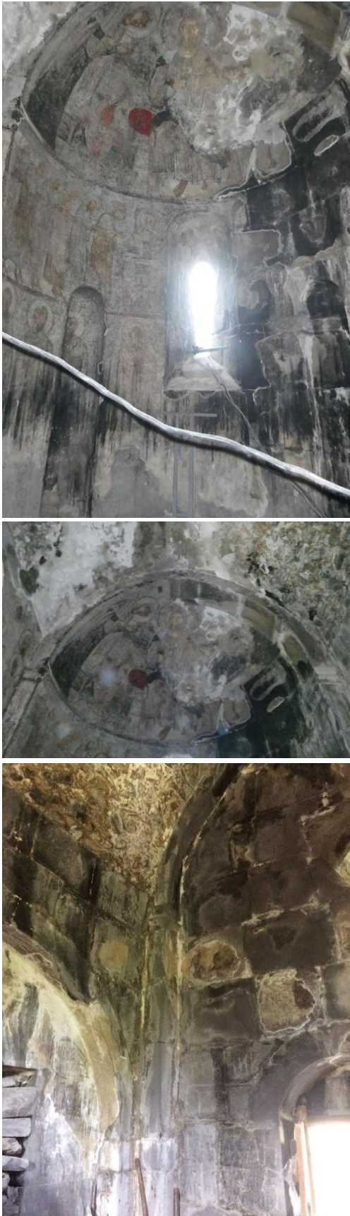
Fig. 3. Due to the poor restoration of the roofing of the Kobayr chapel, as well as the infiltration of rainwater throughout the decades, high-value frescoes of the 12 th century were lost
