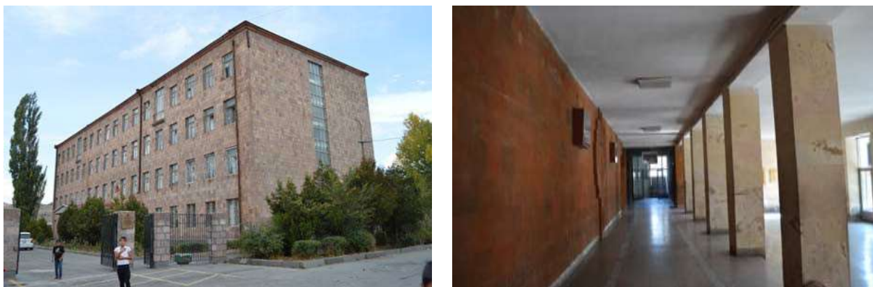
Fig. 1. General and interior views of the building
