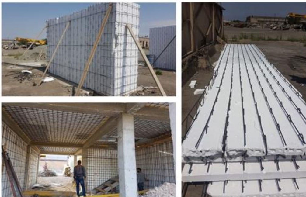
Fig. 2. Three-layer sound- and thermal insulation panels during installation
