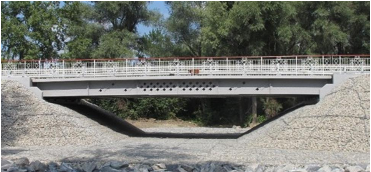
Fig. 1. General view of a bridge with a composite span
