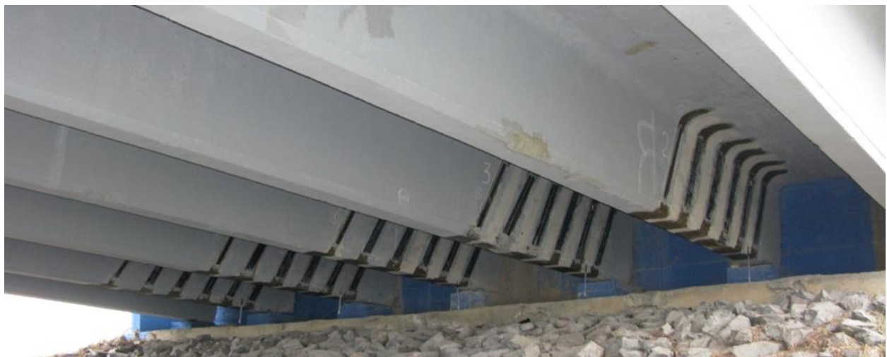
Fig. 4. Bridge beams strengthened in the support section against shear force
