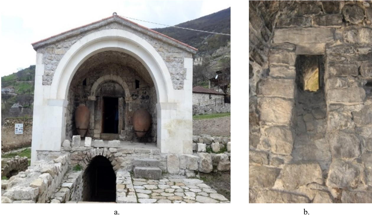
Fig. 8. The northeast facade of the reception area (a): The basement level is accessed through a narrow vaulted corridor. Photo by G.Budaghyan 7 . The small opening of the window (b) expands at a steep angle as it progresses inward. Photo B by M.Titanyan
