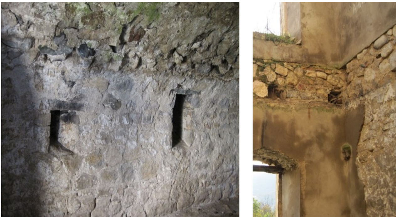
Fig. 12. General view of the "wind-catching" window in the half-floor vaulted room, including the preserved shingle stones. Photo by M. Titanyan
