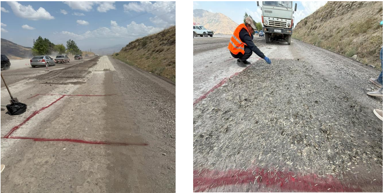
Fig. 3. First and second test sections
