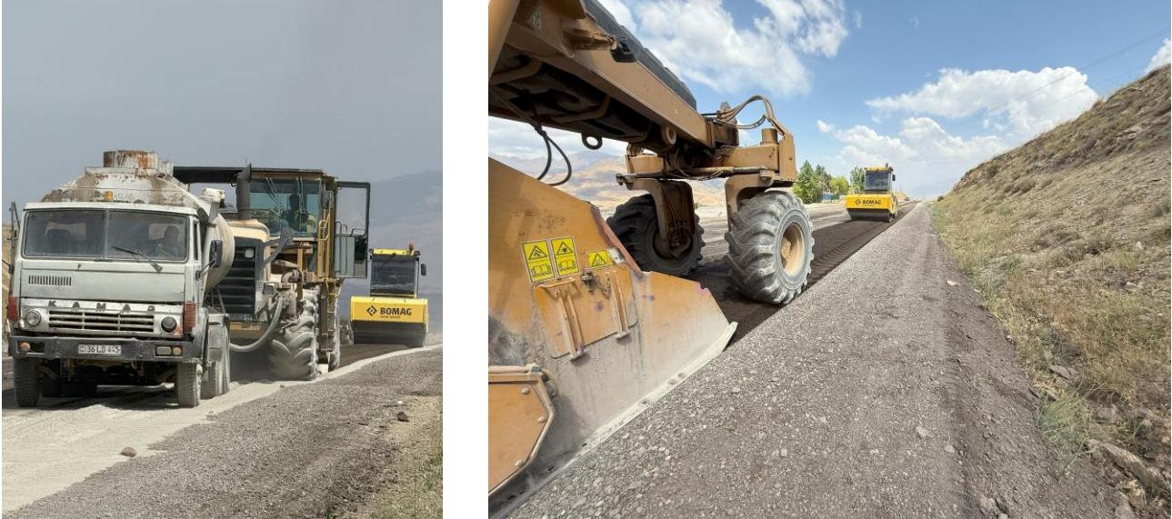
Fig. 5. Full-Depth reclamation and profiling of road pavement
