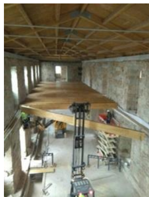
Fig. 9. Timber floors under construction
