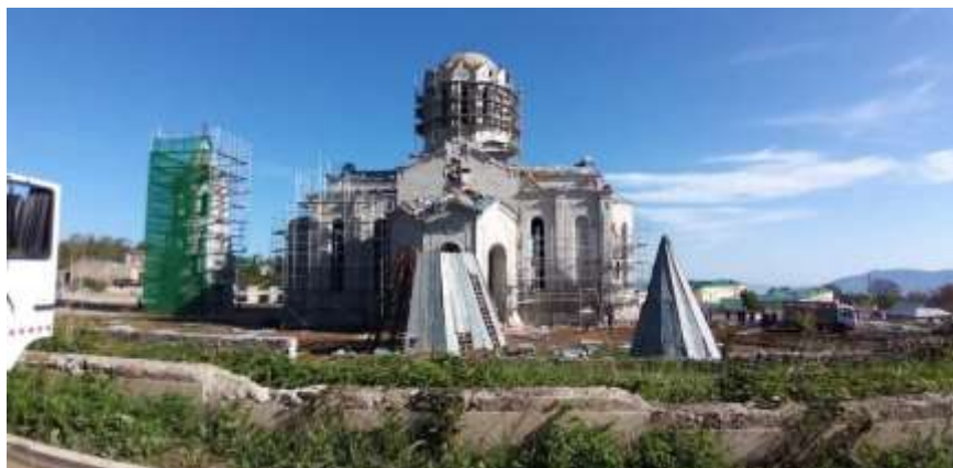
Fig. 14. General view of the of the Holy All Savior Ghazanchetsots Church in Shushi as of 1921
