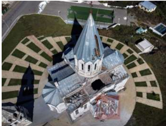
Fig. 13. The condition of the church after the October 8, 2020 missile attack 5
